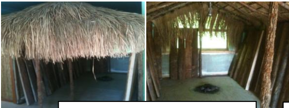
Talai House progressing
